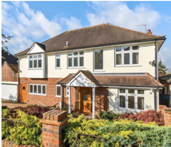
SIX-BEDROOM, DETACHED FAMILY HOME – EPC C Old Park View, Enfield EN2
