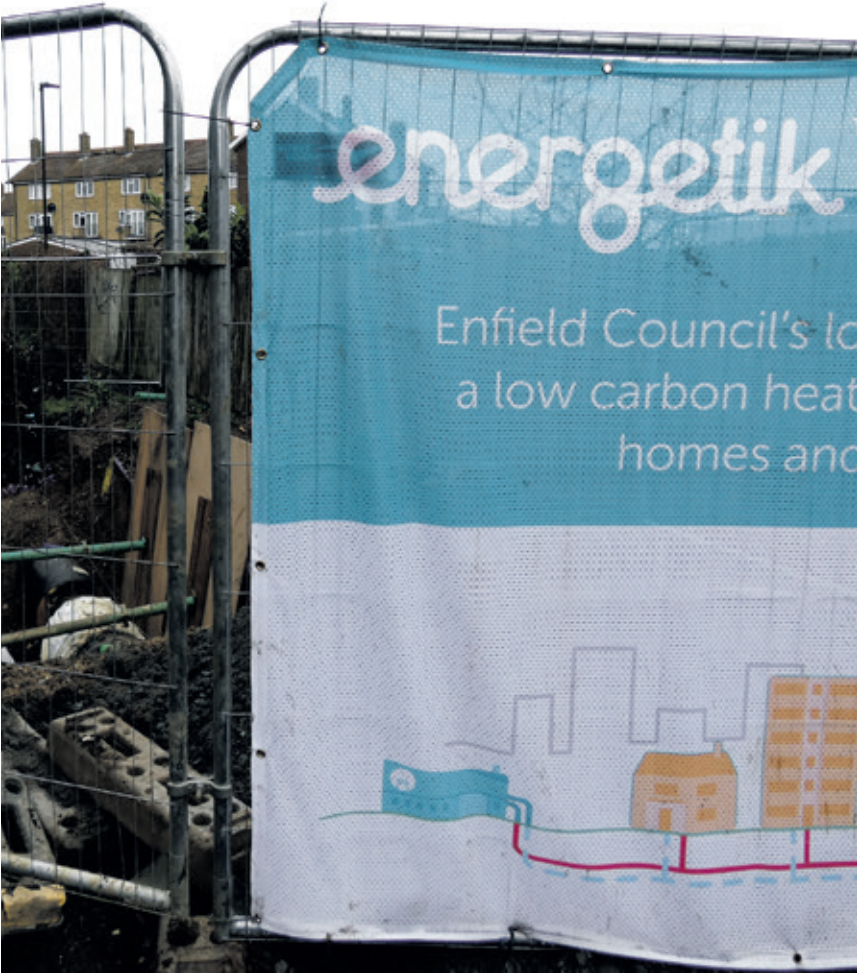
Energetik is already connected to hundreds of Enfield homes but remains under construction
