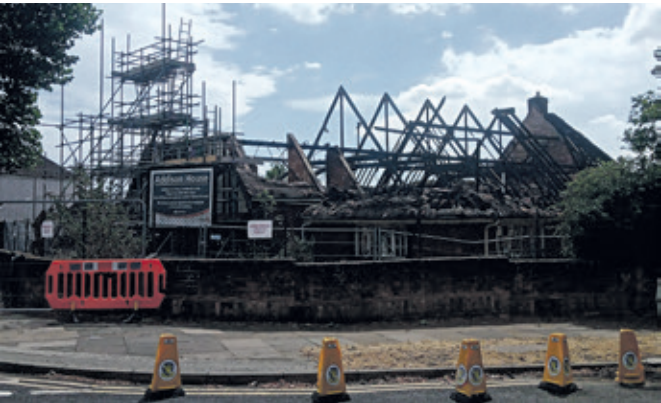
The roof of Addison House was completely destroyed
